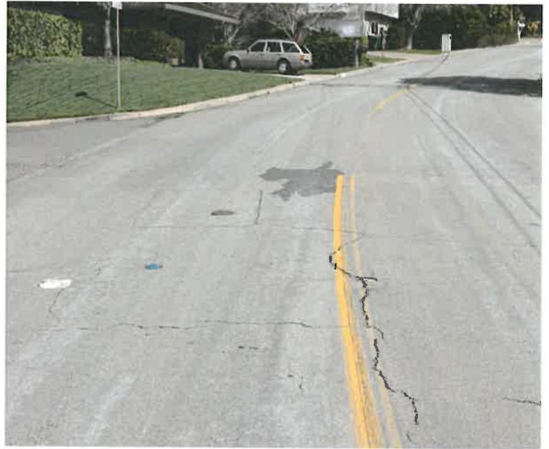
Ardith Drive at Darnby PCI 47
