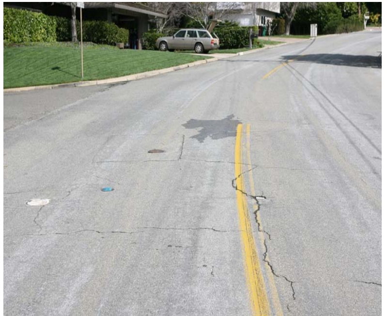
Ardith Drive at Darnby PCI 47
